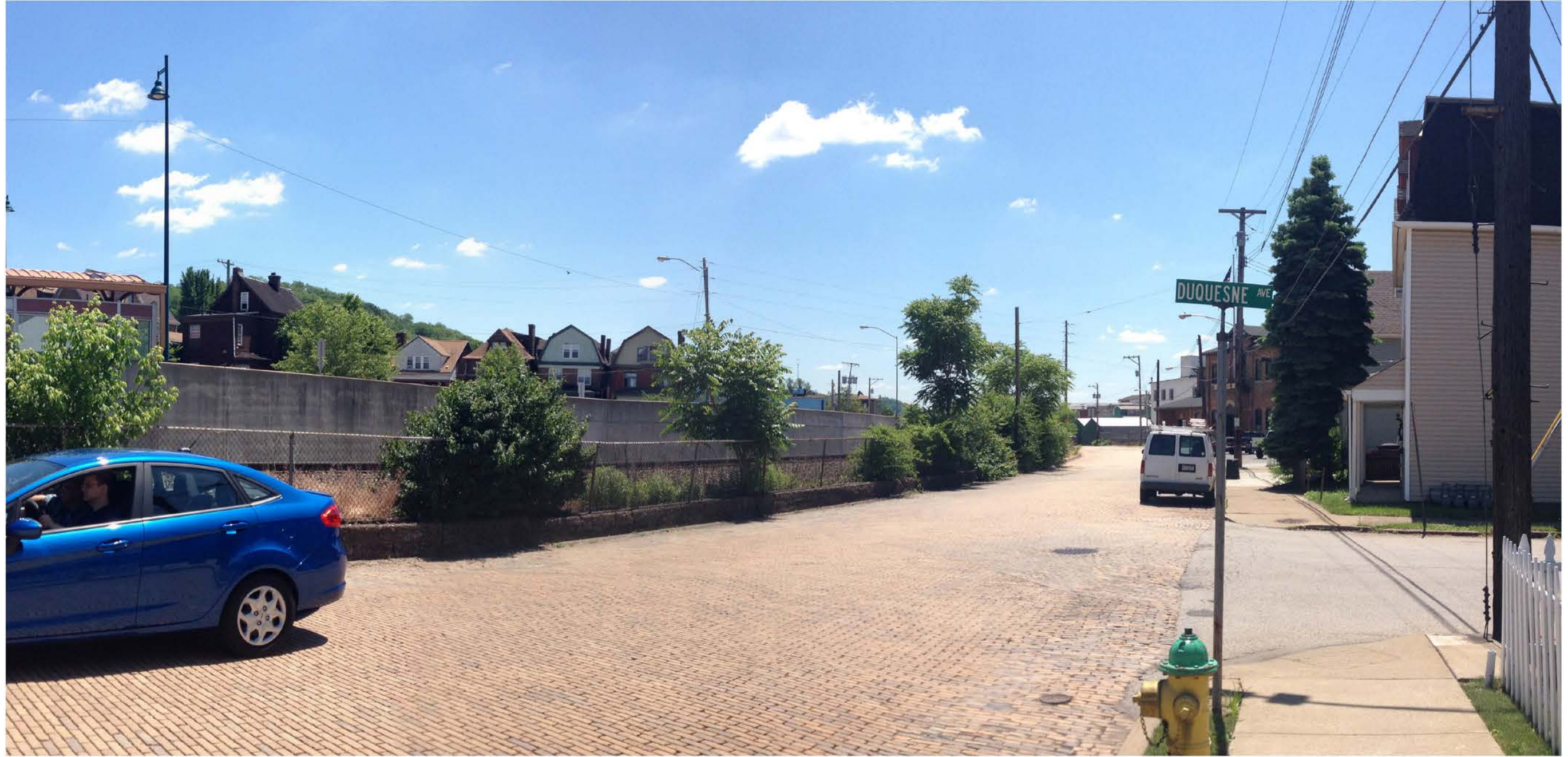
Figure 20 EXISTING CONDITIONS: EAST BUSWAY AT SWISSVALE
