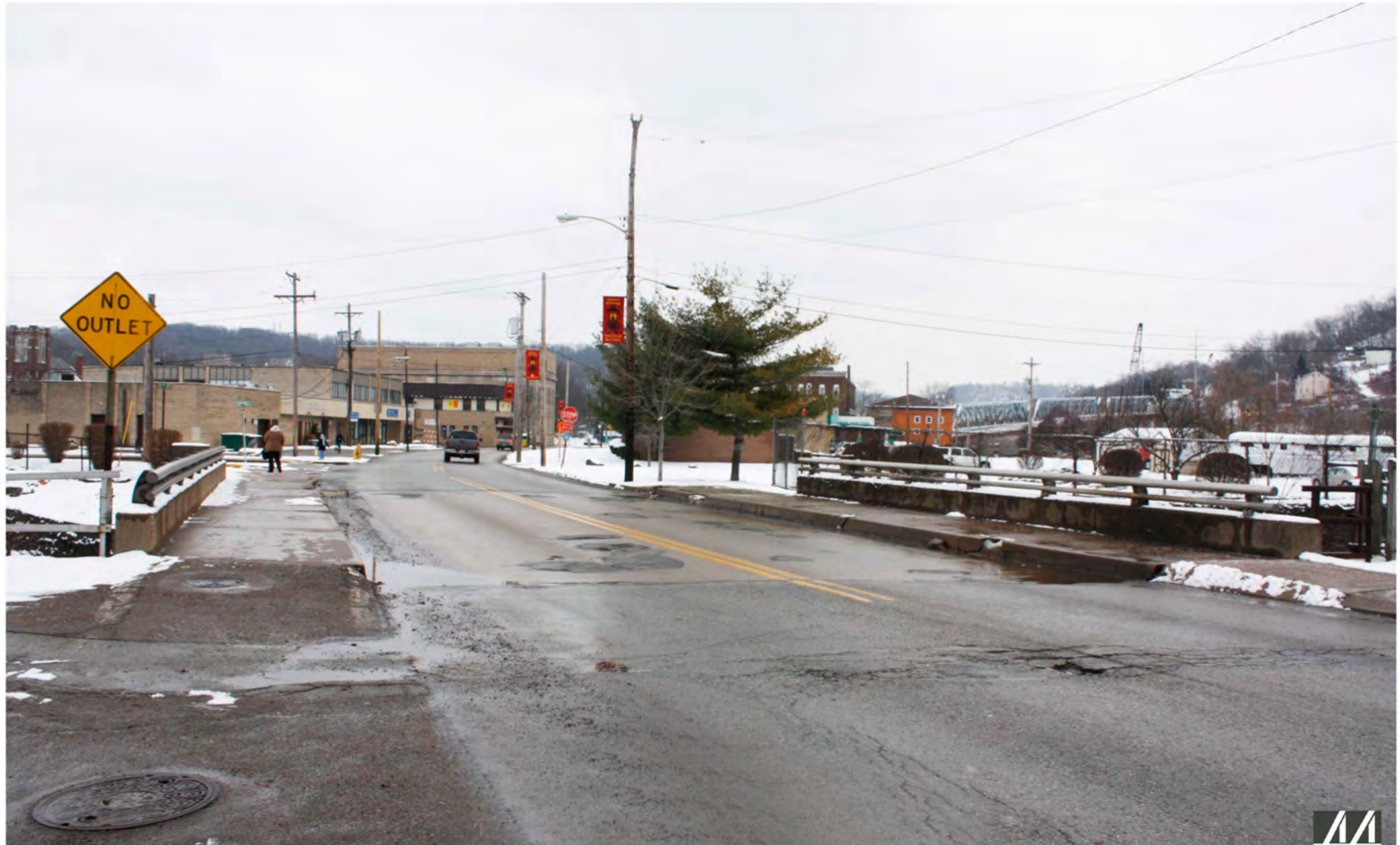
Figure 24 EXISTING PENN AVENUE AT THOMPSON RUN
