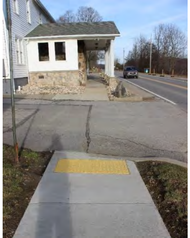
Example of a sidewalk in Hawthorn
