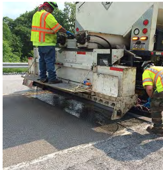
Application of HFST on State Roadway
