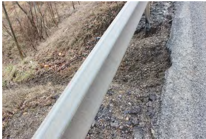
Route 28 between SR 1028 and Lower Hayes Road
