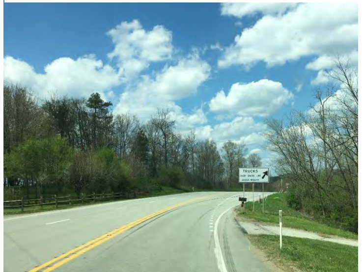
Example of an existing truck brake check area on Route 28
