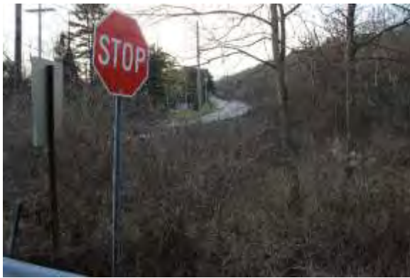
Facing south on Toadtown Road
