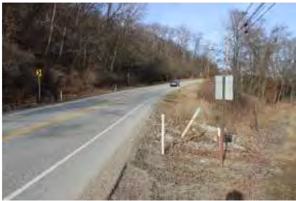
Redbank Valley Trail Crossing, facing north on SR 28
