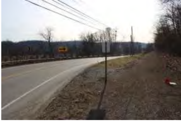
Redbank Valley Trail Crossing, facing south on SR 28
