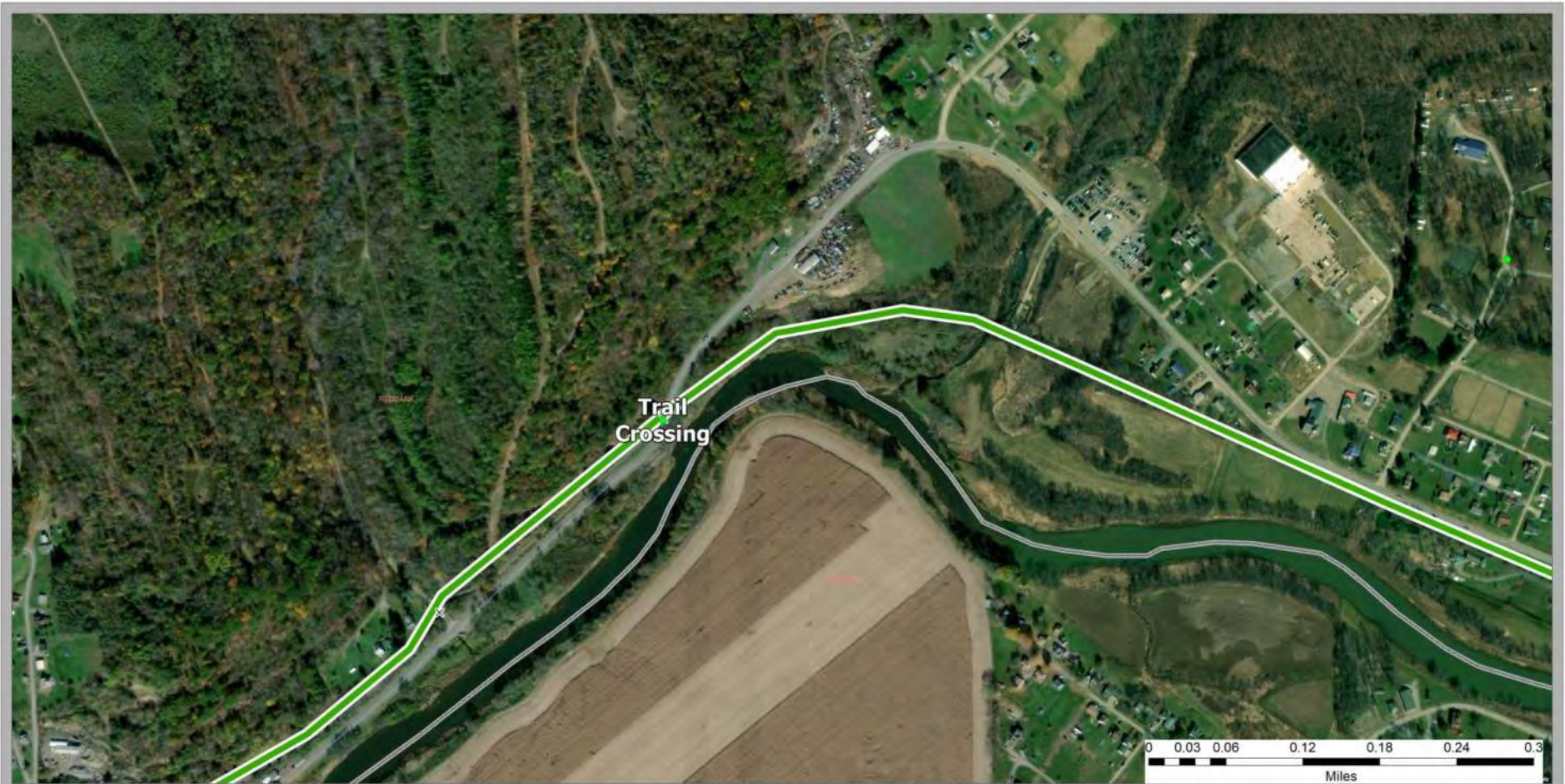
Exhibit 58 - Multimodal Facilities (Redbank Valley Trail Crossing of Route 28)
