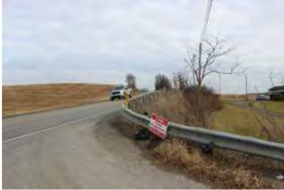
Facing north on SR 28 from SR 1035
