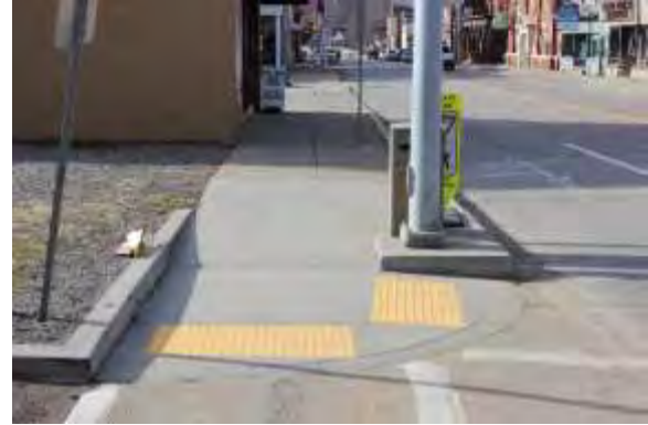
ADA Ramp crossing the entrance from Klingensmith's Drug Store
