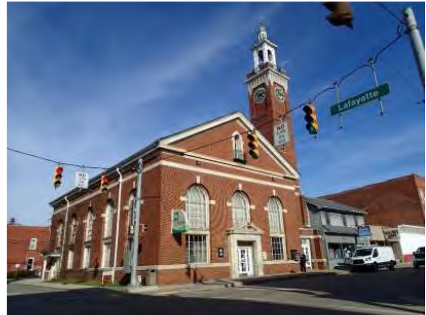
Traffic Signal at Lafayette Street
