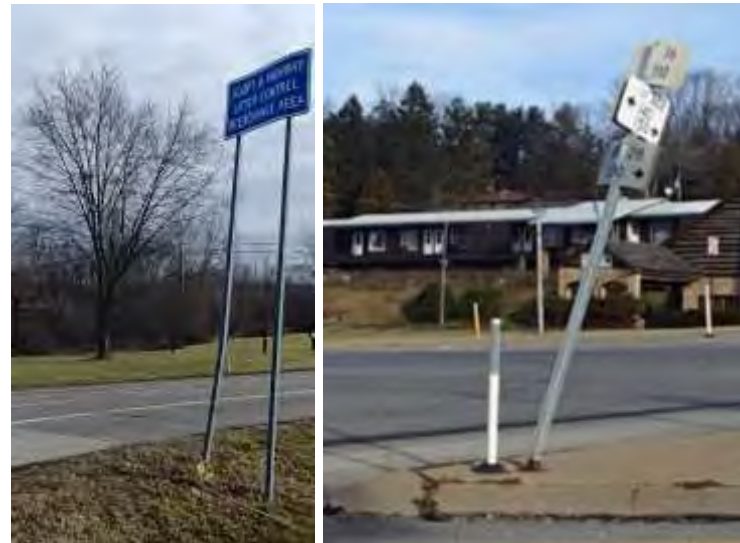
Sign damage at SR 85 and at US 322
