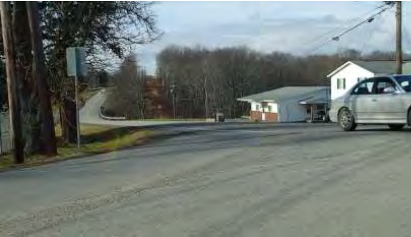
Sight distance looking south at the stop sign on SR 1035
