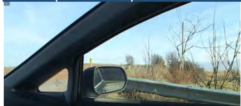
Sight distance limited from crest and guide rail looking north at the stop on SR 1035
