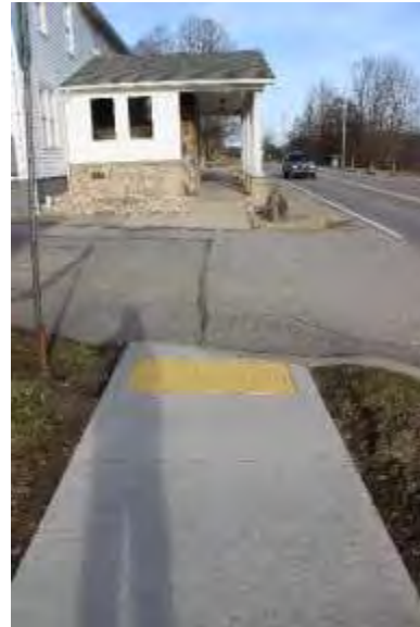
ADA Ramp across from Alcorn Funeral Home at Arch Street
