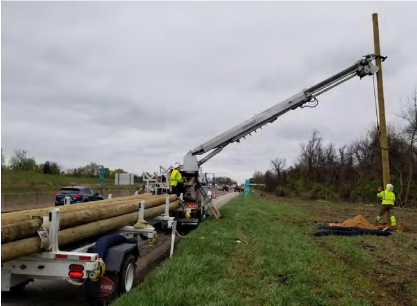
Images from current Eastern Network construction
