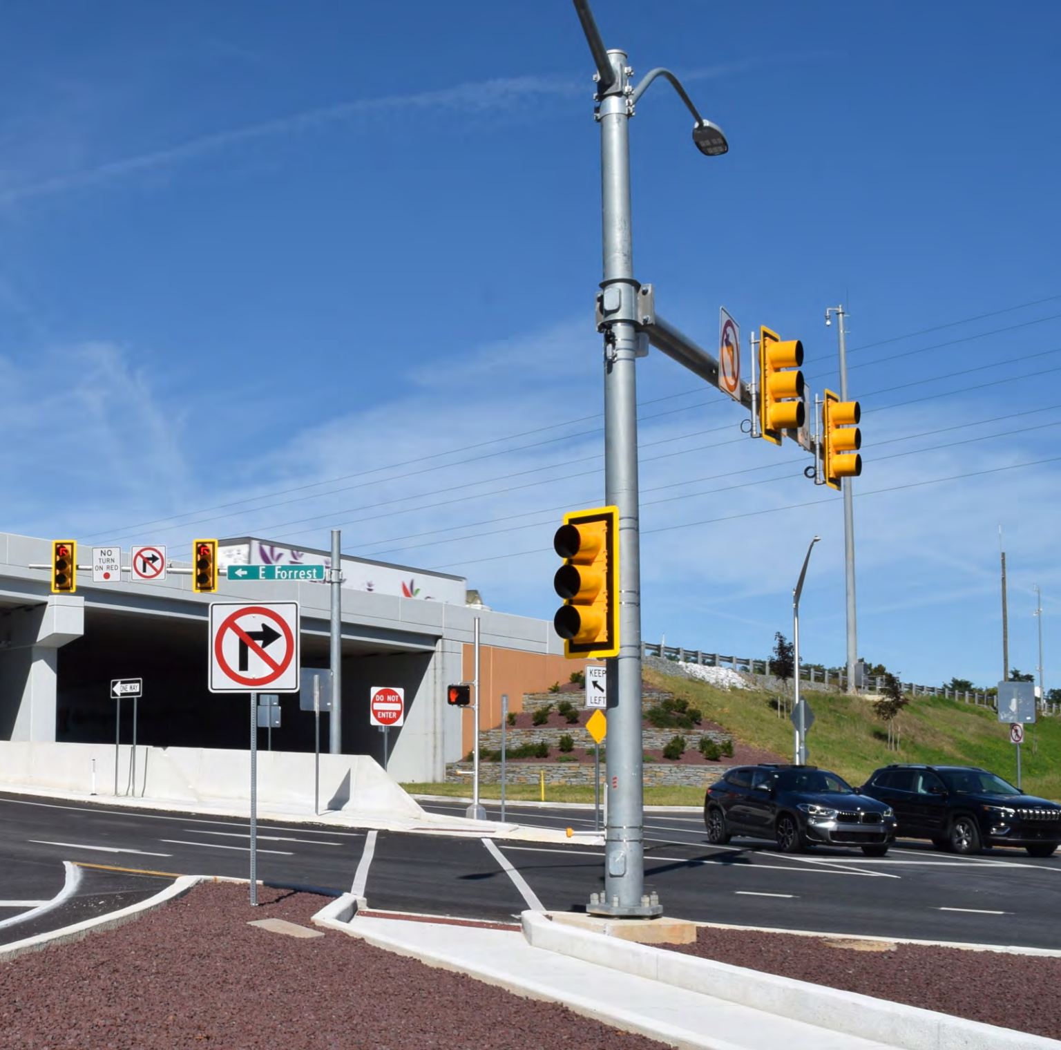
PennDOT is collecting high resolution event logs from Diverging Diamond interchanges for Automated Traffic Signal Performance Measures.
