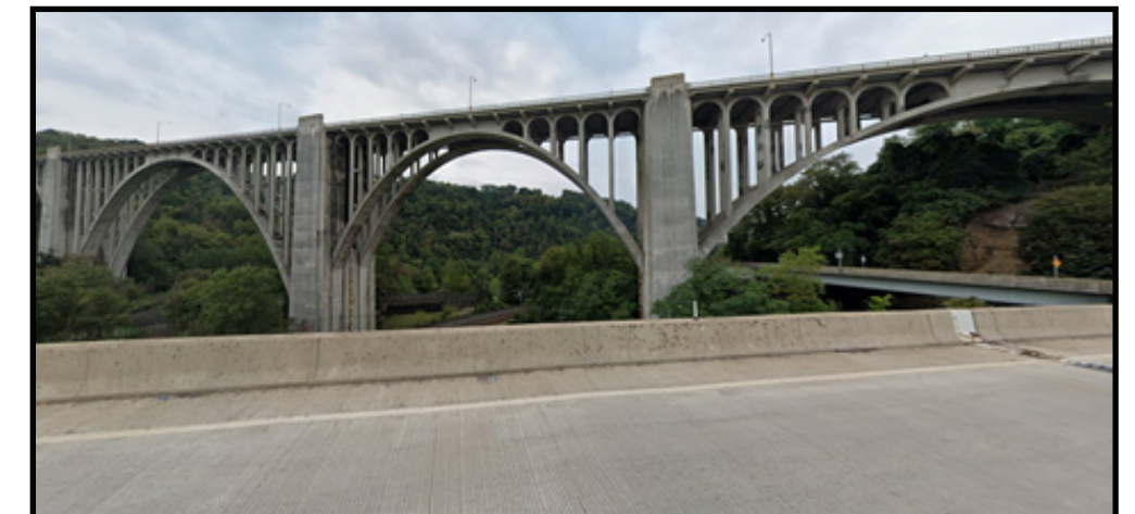
George Westinghouse Bridge
