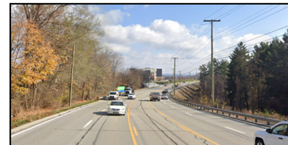
Looking East: US 30 near Little Sewickley Creek.
