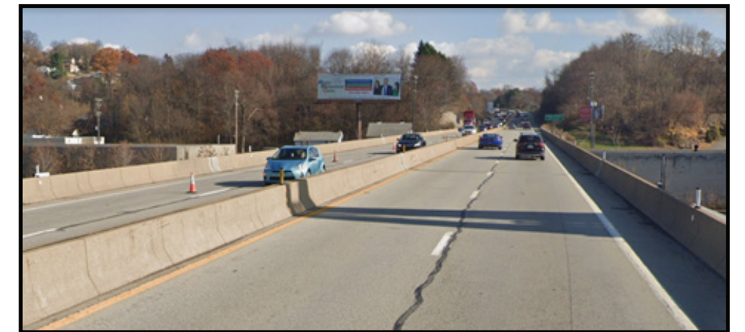
US 30 over Jacks Run (Just east of US 119 interchange)
