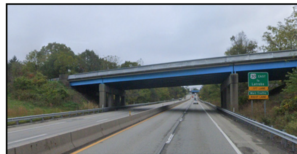
US 30 at SR 130, Hempfield Township
