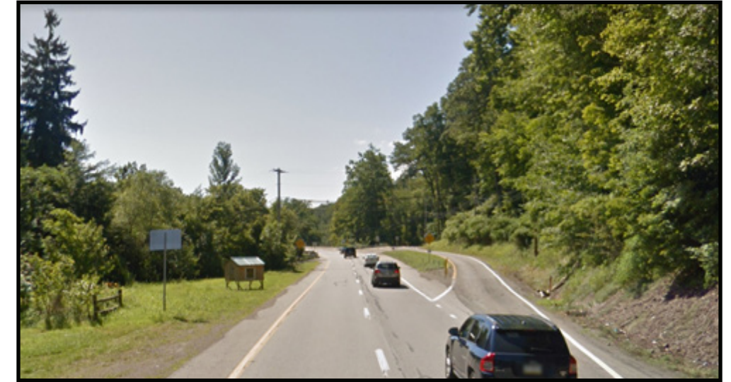
US 30 Eastbound at Darlington Rd
