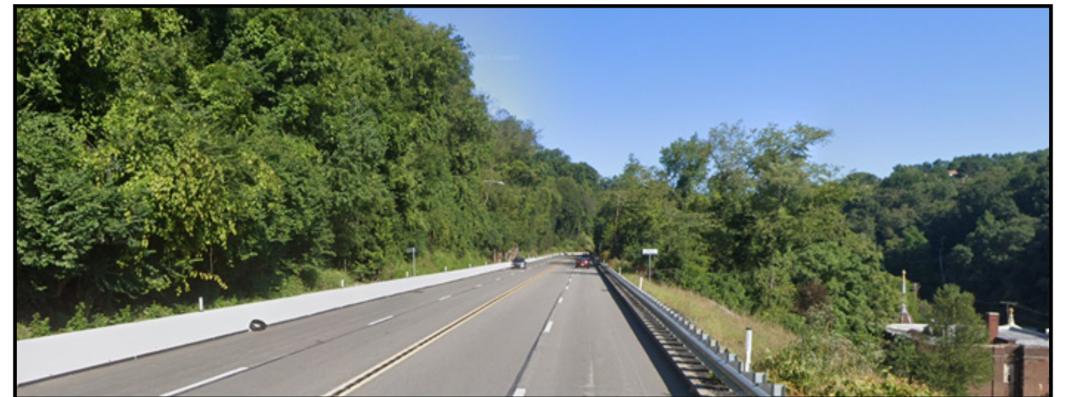
US 30 between Forest Hills and Westinghouse Bridge. This area is highly suceptible to landslides.
