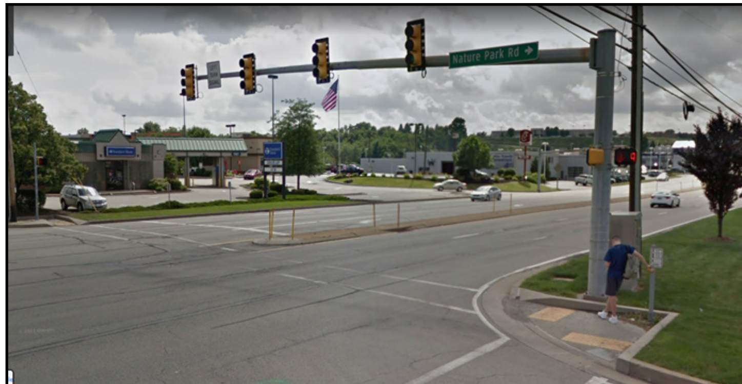
There are pedestrian signals present at the US 30/Nature Park Rd intersection, however, there are no sidewalks present along this section of the corridor.
